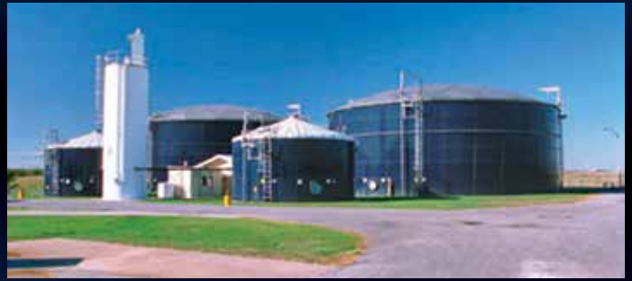
▲ Sludge stabilization and sludge storage facility.
