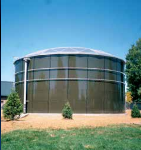
Ground Storage Tank
