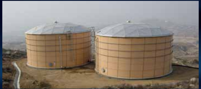
▲ Multiple potable ground storage tank facility.
